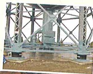
Retrofitted water tank in Seattle, Washington.
