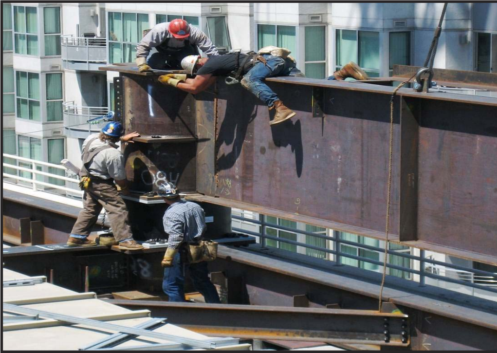
Structural & Seismic Systems Steel: 60' long 6' Plate Girder
