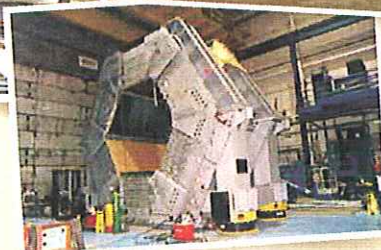
The Stanford Linear Accelerator in Palo Alto, California is protected by DIS isolators.
