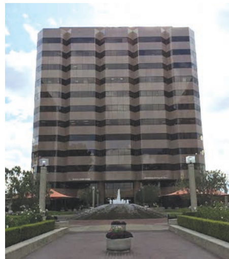
MetroCenter: fountain to make way for food truck runway, other amenities
