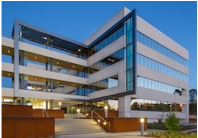
Enclave Sorrento after renovation
